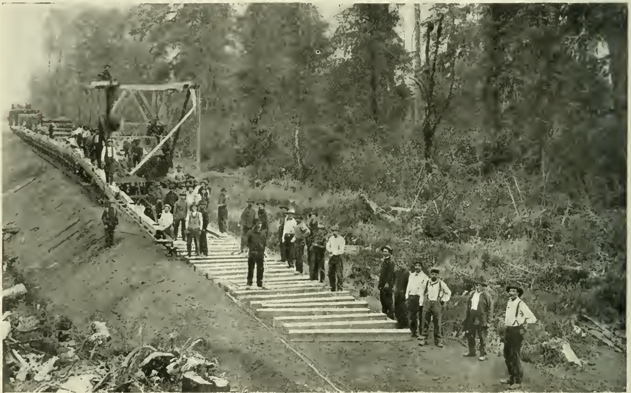
TRACK LAYING IN THE WOODS.
